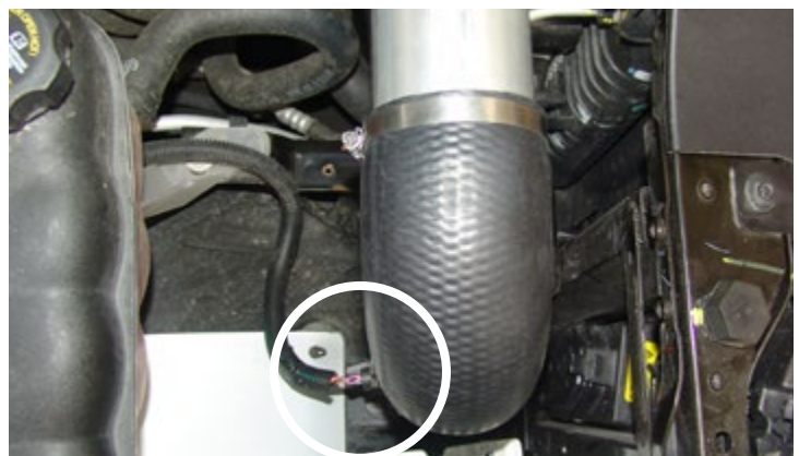
MAF Electrical Connection
