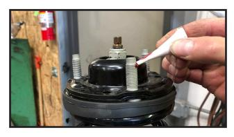
11. Locate Stud extenders in the hardware bag. Install them onto the top hat studs and tighten.
