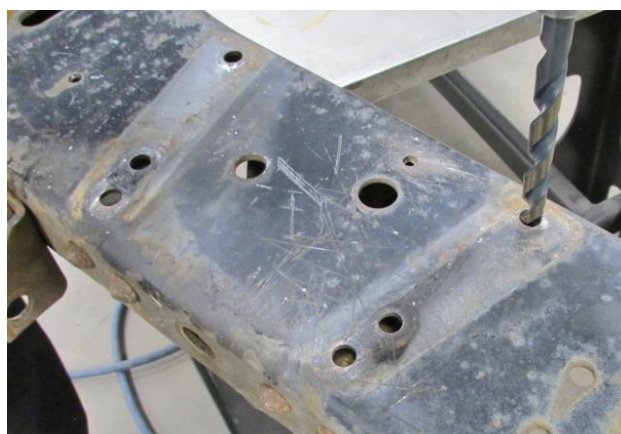
Figure 17 - Drill Out Frame Holes
