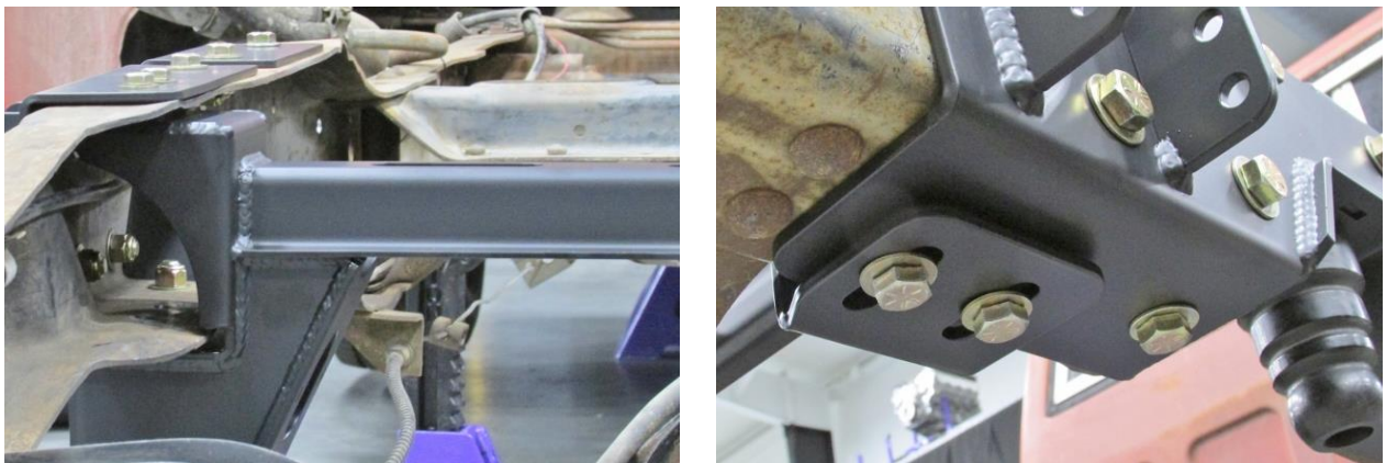
Figure 14 - Install Track Bar Crossmember
