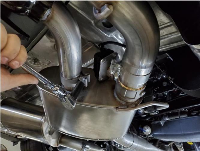
**21. (S.S. TIPS ONLY)** Snugly tighten the clamp securing the inner tip assembly to the muffler using a 15mm deep socket and 3/8" ratchet, leaving it loose enough for later adjustment. Repeat **INSTALL STEPS 18-21** for the driver side inner tip assembly.
