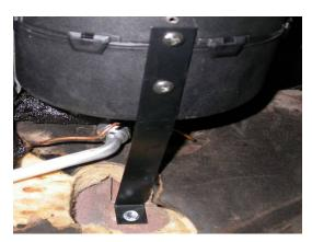
Install the blower support brace, as shown using (2) #8 x 3/8" screws, and (1) #10 x 3/4" Tek screw.
