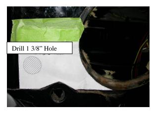
Locate blower motor service hole on the firewall. Using Template supplied, cut out and locate on firewall as shown. Drill a 1 3/8" hole through firewall.
