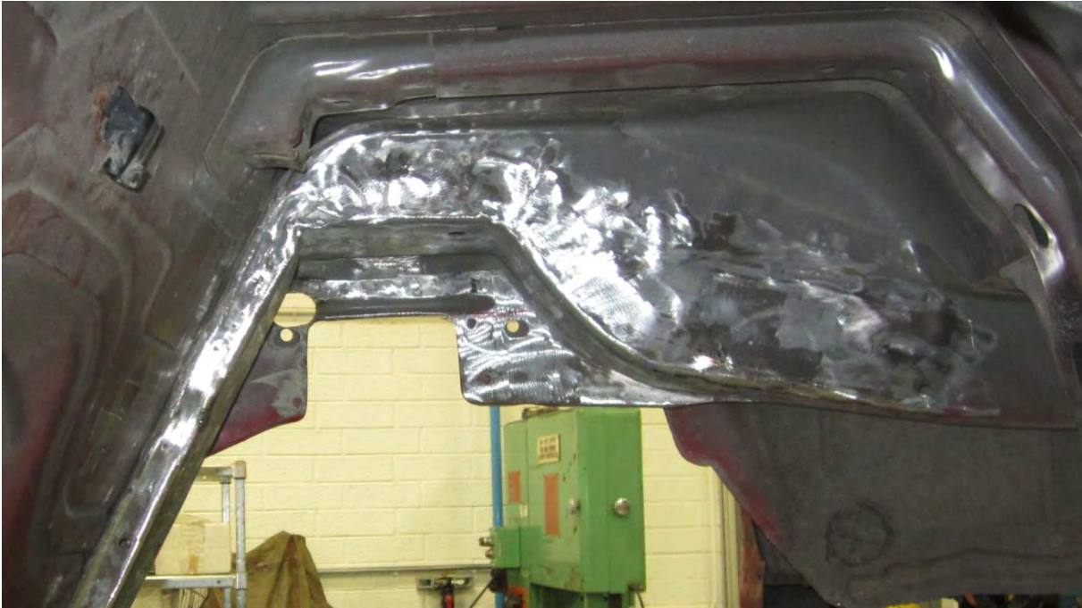
Inside View, Passenger Side Frame Rail, Figure 18
